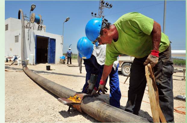
Training Center Ability to test new advances in grid and metering technology
